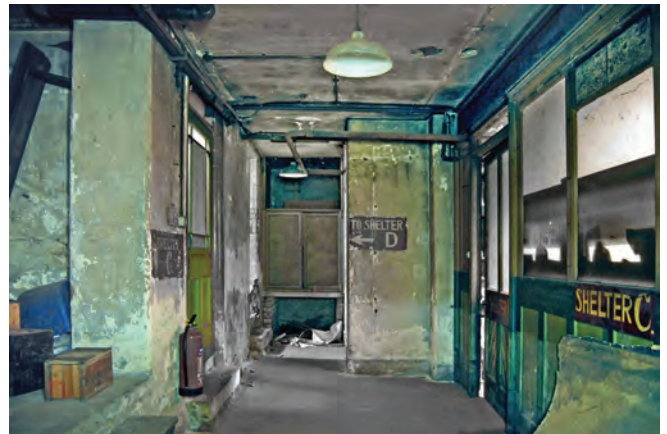
The well-meaning owners of this Leeds factory provided a comfortable and well-appointed shelter for their staff but without basic ARP protection this could have been a death-trap like many other factory basement shelters
